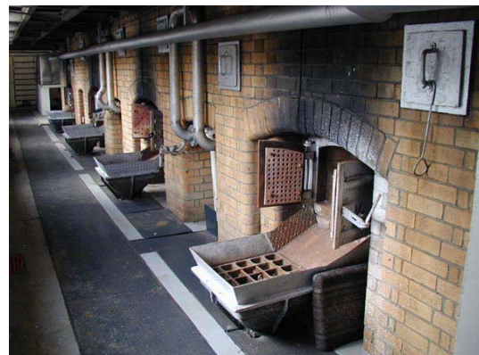
The old coal-fired furnaces in distillery
